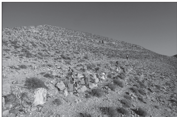
10. Retaining wall of the ancient road, west of Boz al-Mushelle, looking east.
